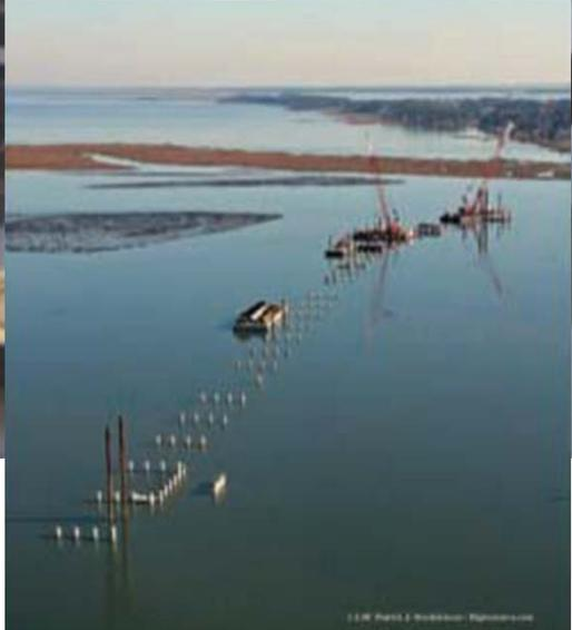
Fifty-four piles were driven below the mud line for the bascule footing. Piles were driven inside a cofferdam and are typically driven in pier bents within a template frame. Bents ranged from three to five piles each. American Bridge expects to complete the project on time in November 2009.
