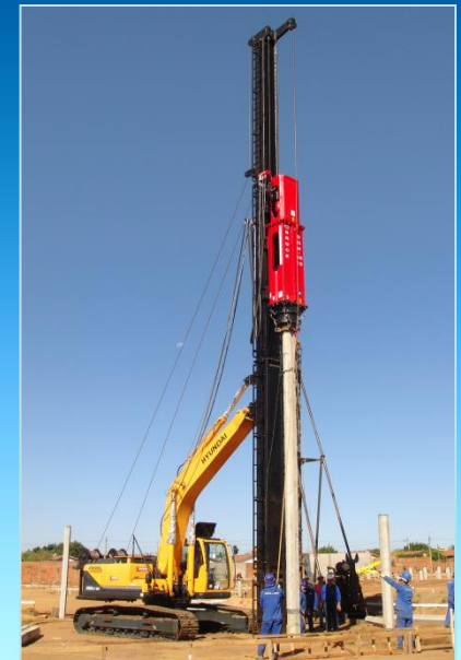
Excavator Mounted Hammer
