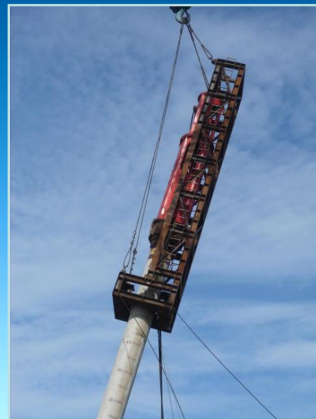
Batter Pile Driving Crane Suspended Leader
