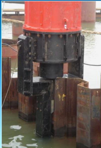
Steel Sheet Pile
