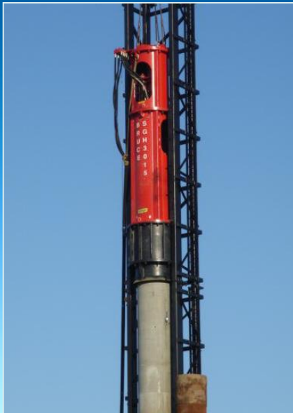
Rounded Concrete Pile
