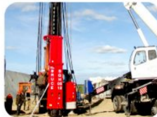
7) Set up a Hammer with Sheave
