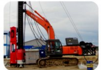
8) Ready for the work
