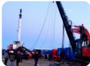
6) Connect the Winch Wires
