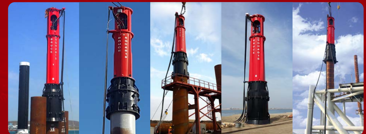
Hammers working with crane suspended type.
