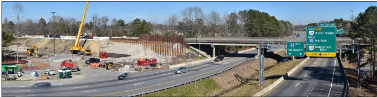
Current View of Great Bridge Blvd Bridge (Looking West)
