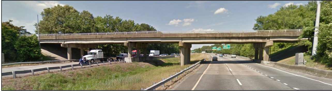
Existing Great Bridge Blvd Bridge (Looking East)
