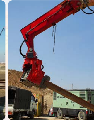
Lift the pile
