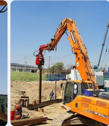
Drive the pile
