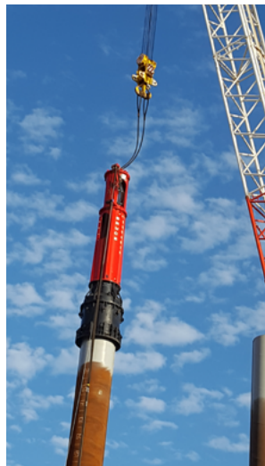
Hammers working with crane suspended type.
