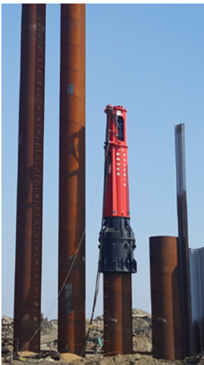
Hammers working with crane suspended type.
