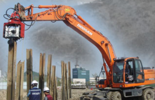
EXCAVATOR MOUNTED VIBRO
